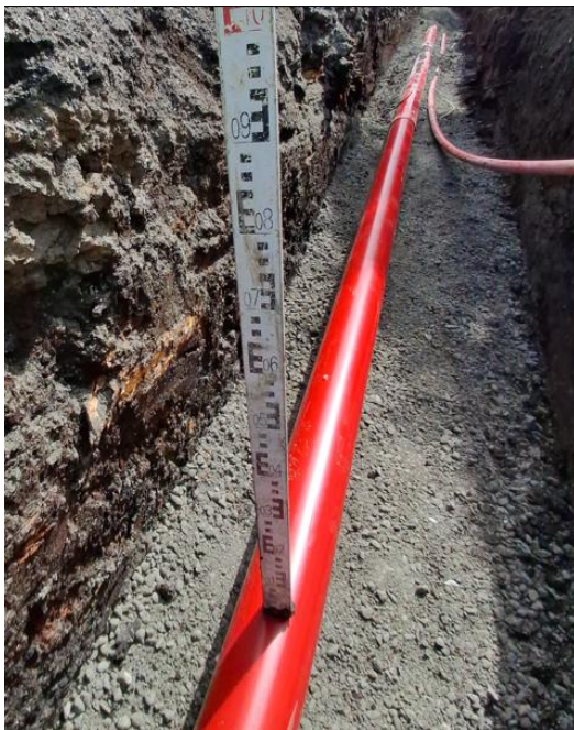
Plate 2-1 Typical Single Cable Trench View
