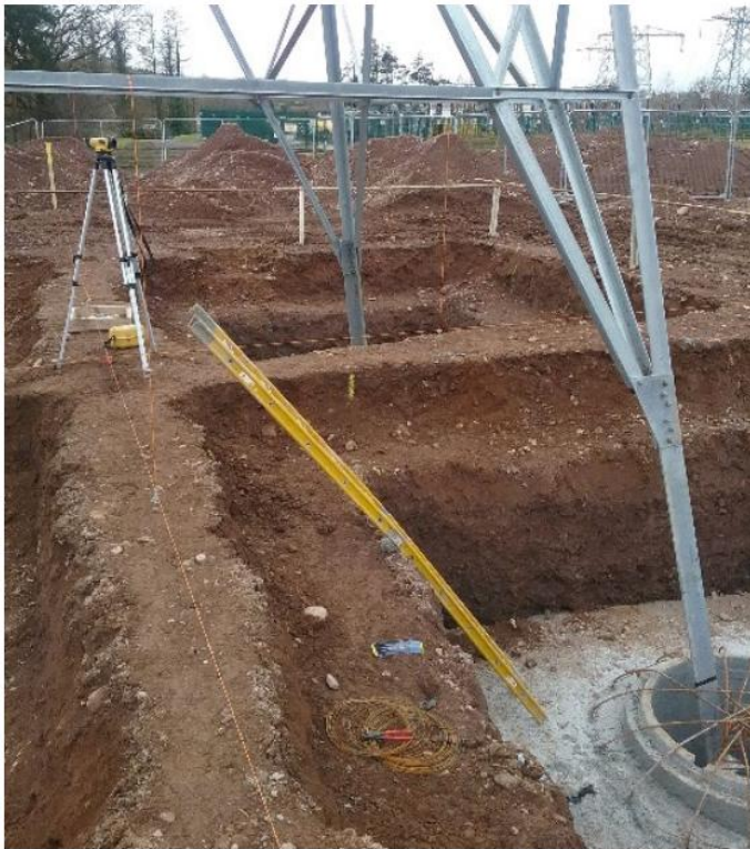
Plate 2-9 Typical 110kV end mast foundation excavation (example image)
