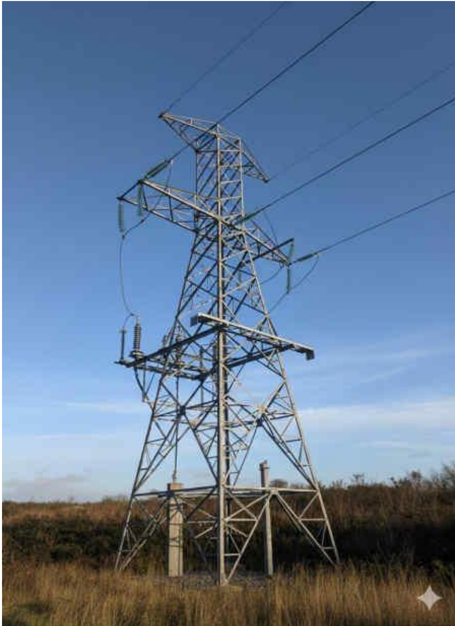
Plate 2-12 Cable end mast
