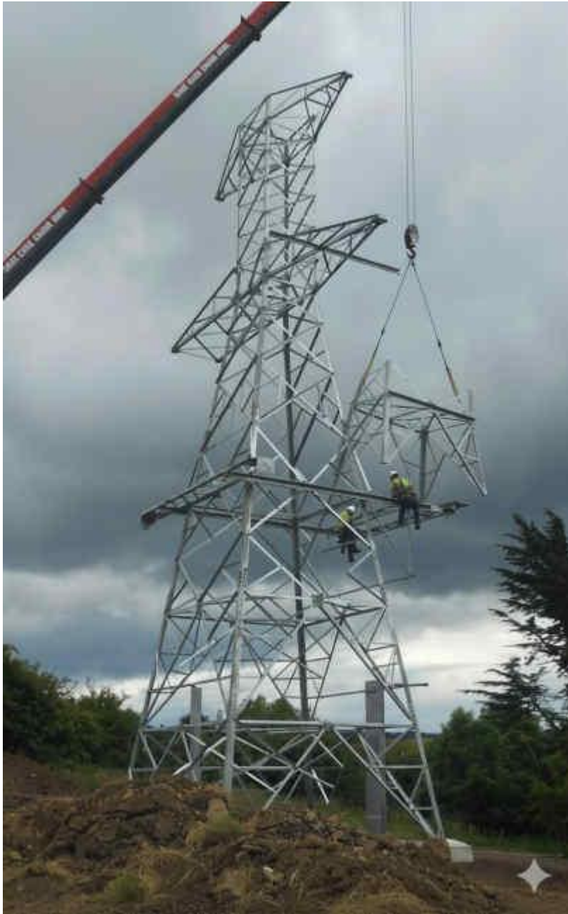
Plate 2-11 End Mast under construction
