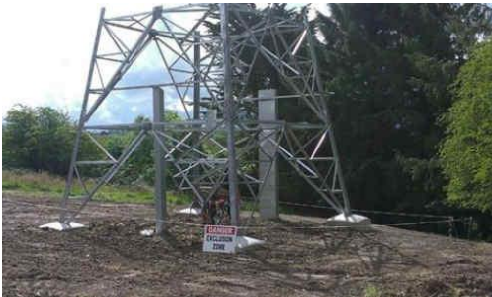
Plate 2-10 Base of end mast structure backfilled
