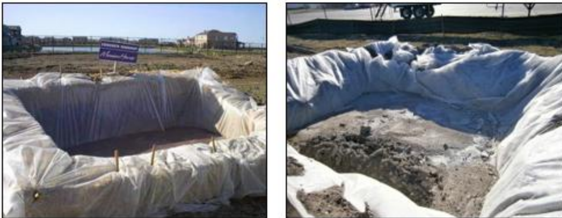
Plate 3-2 Typical concrete wash out areas
