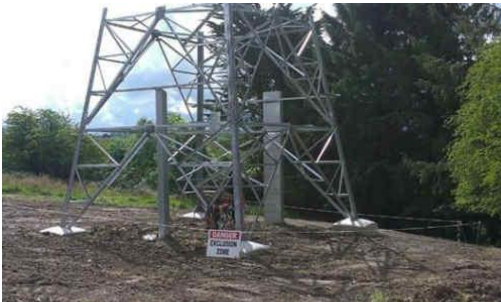
Plate 2-10 Base of end mast structure backfilled
