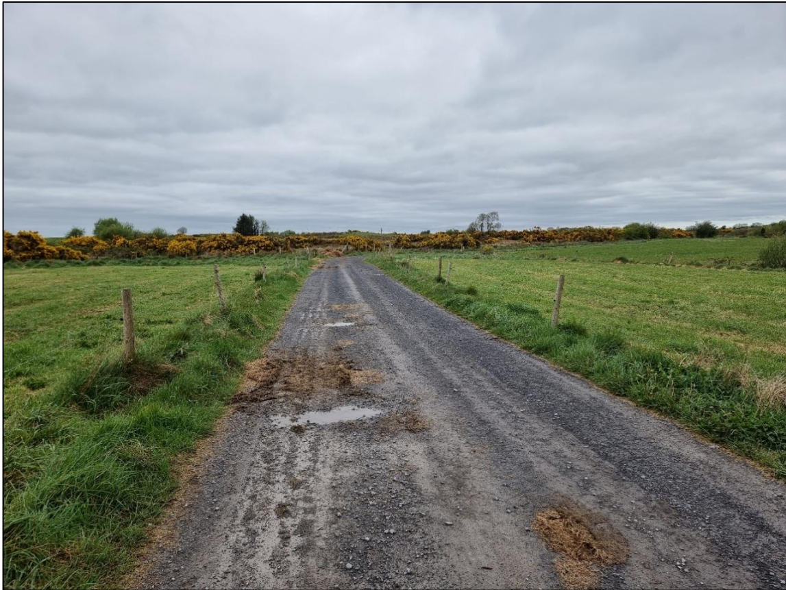
Plate 6-35 Main access road to the Site (L15053), classified as Buildings and artificial surfaces (BL3)
