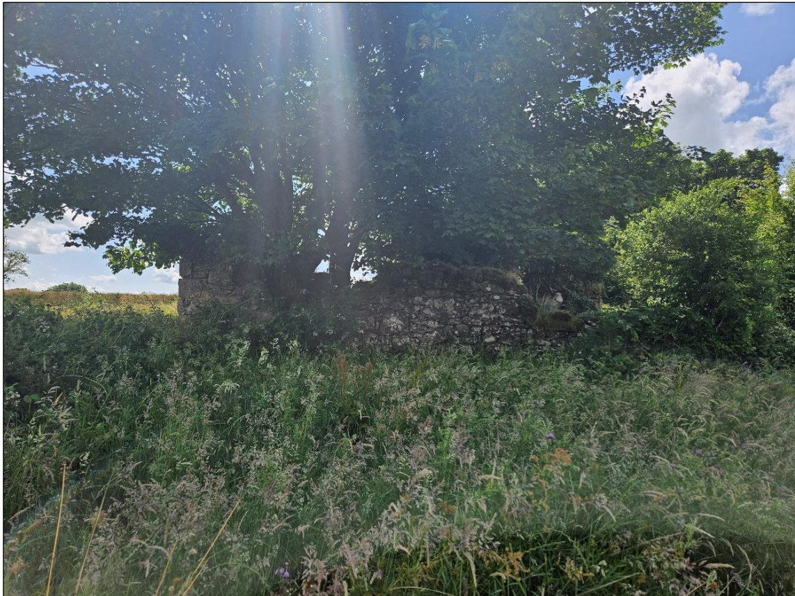
Plate 6-34 Old stone building classified as Stonewalls and other stonework (BL1) located at the southeast of the Site.
